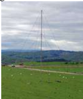
PIC: Cubra Stratton mast as installed at Quartz Hill.
