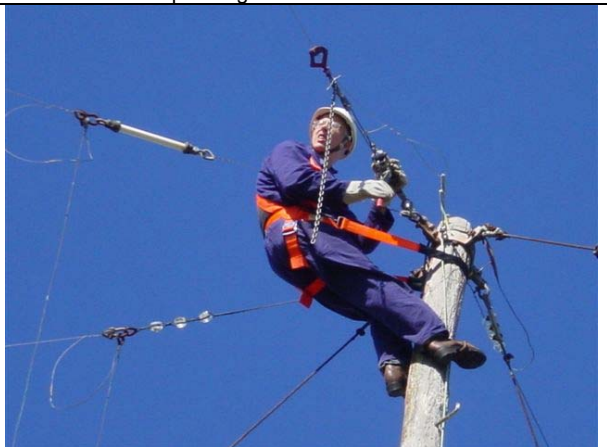
Brian ZL1AZE doing antenna maintenance atop one of the 20-metre masts
