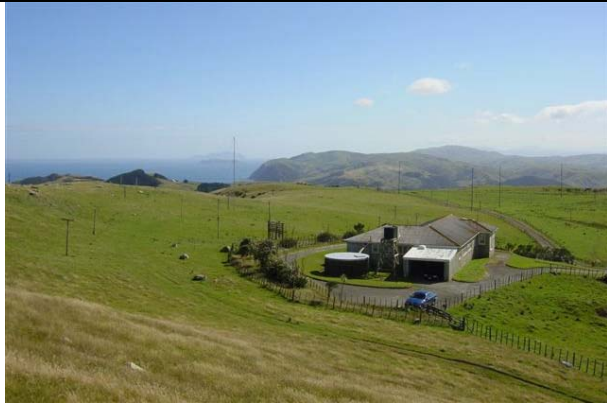
View looking north across the main building towards Mana and Kapiti Islands
